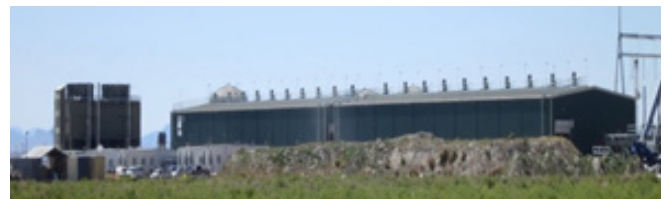
The ACES Delta site where Mitsubishi subsidiary MHI Hydrogen Infrastructure plans to make green hydrogen to supply the IPP gas plants. Mitsubishi anticipates the electrolyzer facility will create 20 permanent jobs, some of which have already been filled by former IPP employees.
