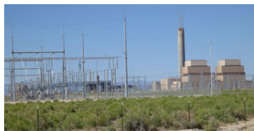
The IMP Project on the outskirts of Delta, a small town of roughly 4,000 residents in Utah's West Desert.
